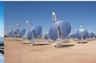
Parabolic dishes with Stirling <sup>12</sup> motors
