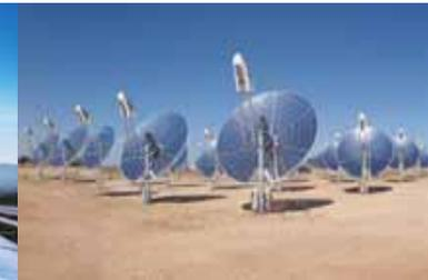
Parabolic dishes with Stirling motors
